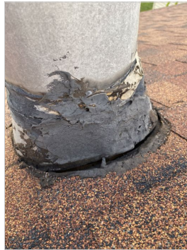
Furnace Roof Vent
