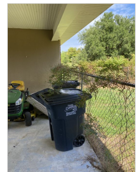
Possible toxic vegetation extended into walking path outside exterior door.
