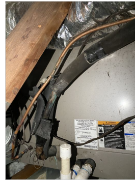
Missing Insulation
