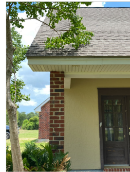
Front northwest corner has vegetation on roof.
