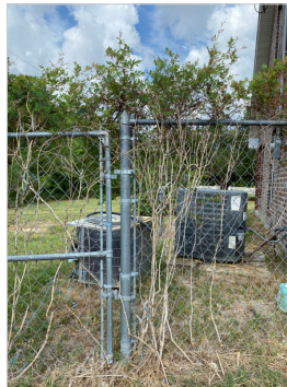
Gate not able to move due to vegetation growth.
