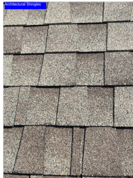
Weathered Wood Architectural Shingles
