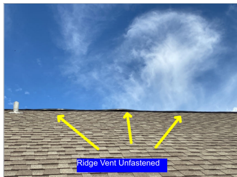
Ridge vent should be fastened to prevent pest and moisture intrusion to attic.
