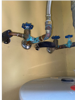
Previous tubing connections to outside condenser.
