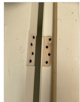
Rear Entry Door missing hinge.
