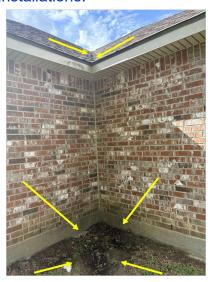
Soil washed away against foundation due to roof Soil washed away against foundation due to roof valley water drainage.
