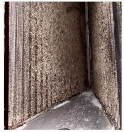
Evaporator was clogged due to incorrect filter design.
