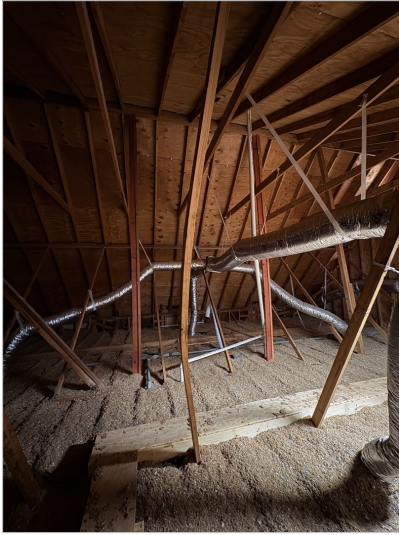
Warped purling support board.
