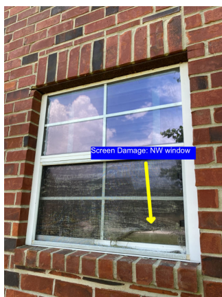
Northwest Window: Screen damage.
