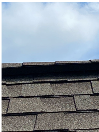
Ridge vent should be fastened to prevent pest and moisture intrusion to attic.
