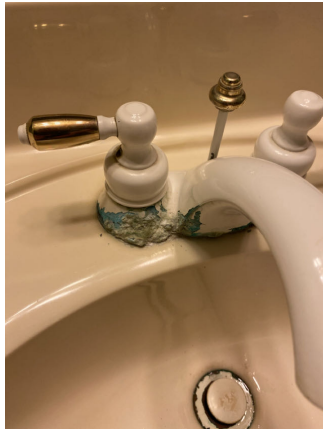
Upstairs Bath faucet leaking and corroded.
