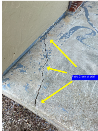
Front Patio: North end of lateral crack.
