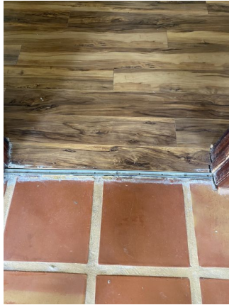
Transition strip is missing between master bedroom and living room.
