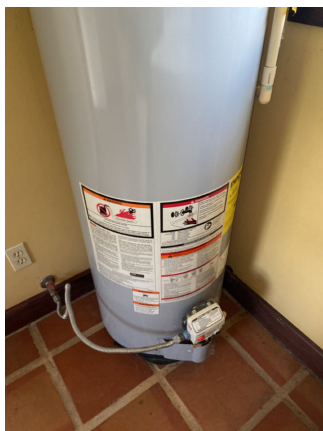
Gas Water Heater - No drip pan installed.
