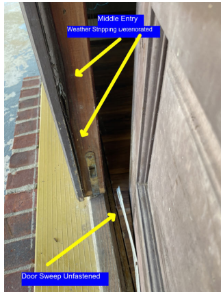
Middle Entry Door weather stripping damage and unfastened door-sweep.
