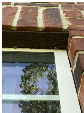
No seal. Lintel rusted.
