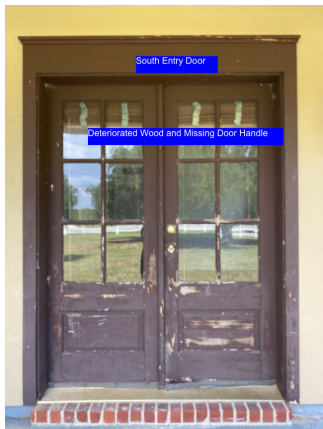
South Entry Door: Coating deteriorated, missing handle.
