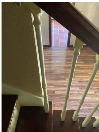
Balusters were spaced more than 4".
