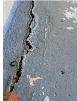
Crack along the wall.
